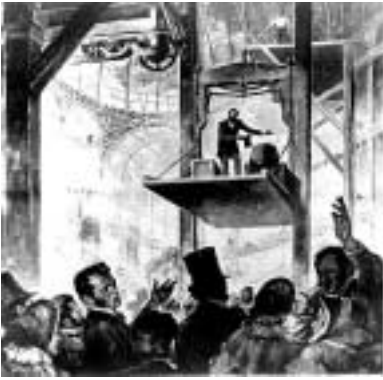
Fig. 4.4.3 - The modern era of elevators began in 1853, when Elisha Otis first demonstrated his Safety Elevator. He stood in the elevator car, high above the ground, while an assistant cut the rope that supported it. A mechanism in the car immediately grabbed onto the side rails and prevented the car from falling.
