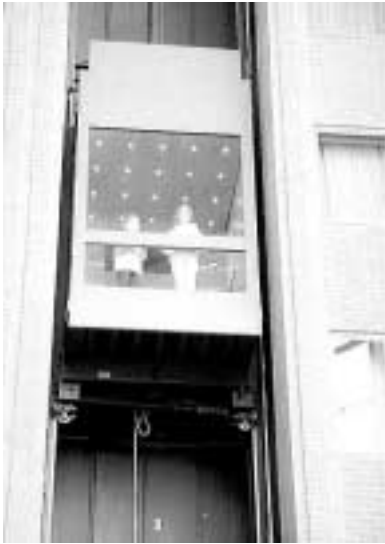
Fig. 4.4.7 - The car of this elevator is pulled upward from above by 4 cables and rides on rails to its left and right. The riders control the car through the electric cable hanging below the car.
