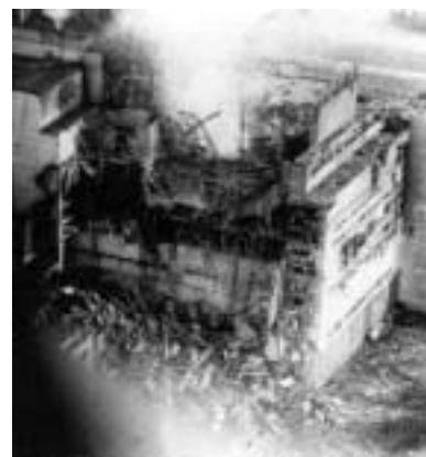
Fig. 14.3.5 - Several hours after a misguided experiment caused it to exceed critical mass and vaporize parts of its core, Chernobyl Reactor Number 4 continues to emit radioactive smoke and steam.
