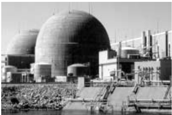
Fig. 14.3.4 - The North Anna Nuclear Power Station in Mineral, Virginia uses two Westinghouse pressurized light water reactors to generate a total of 1900 MW of electric power. At capacity, each reactor produces more than 2,900 MW of thermal power and can generate 950 MW of electric power. Waste heat from the plant is deposited in nearby Lake Anna.
